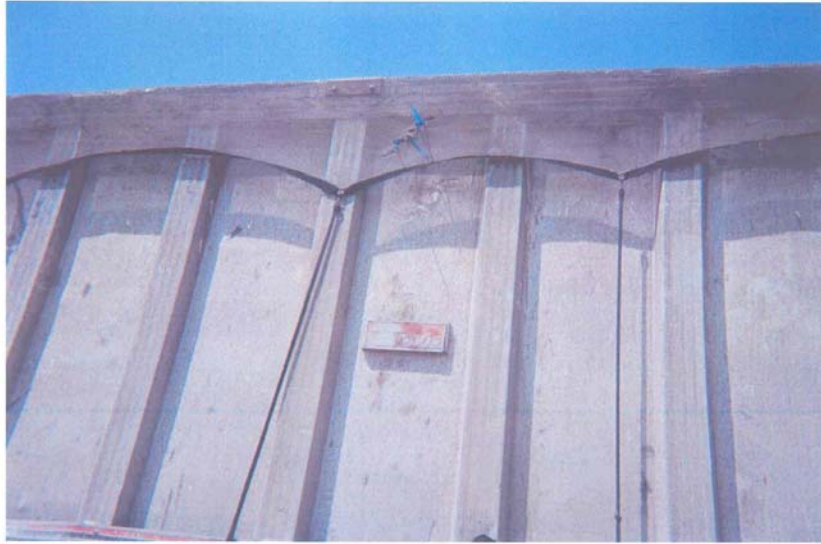
Photo No. 5: Proper repair of torn mesh cover.
